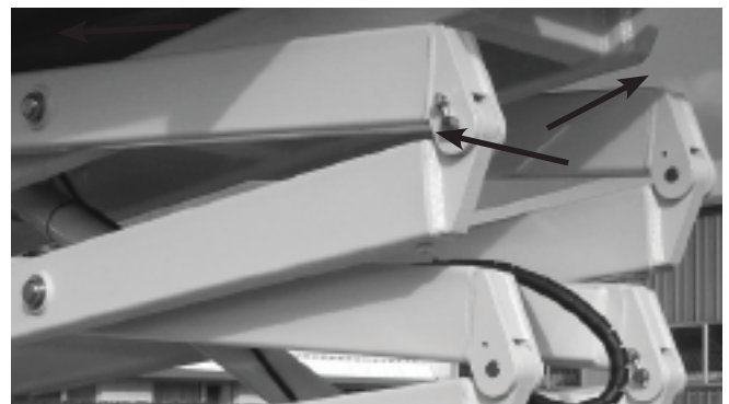
Figure 7.19 - Structural Damage and Welds
